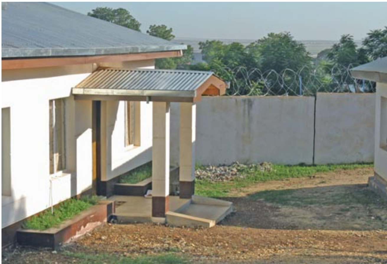
Figure 2. UNHCR residential compound, Juba, South Sudan. Photo: Mark Duffield.
