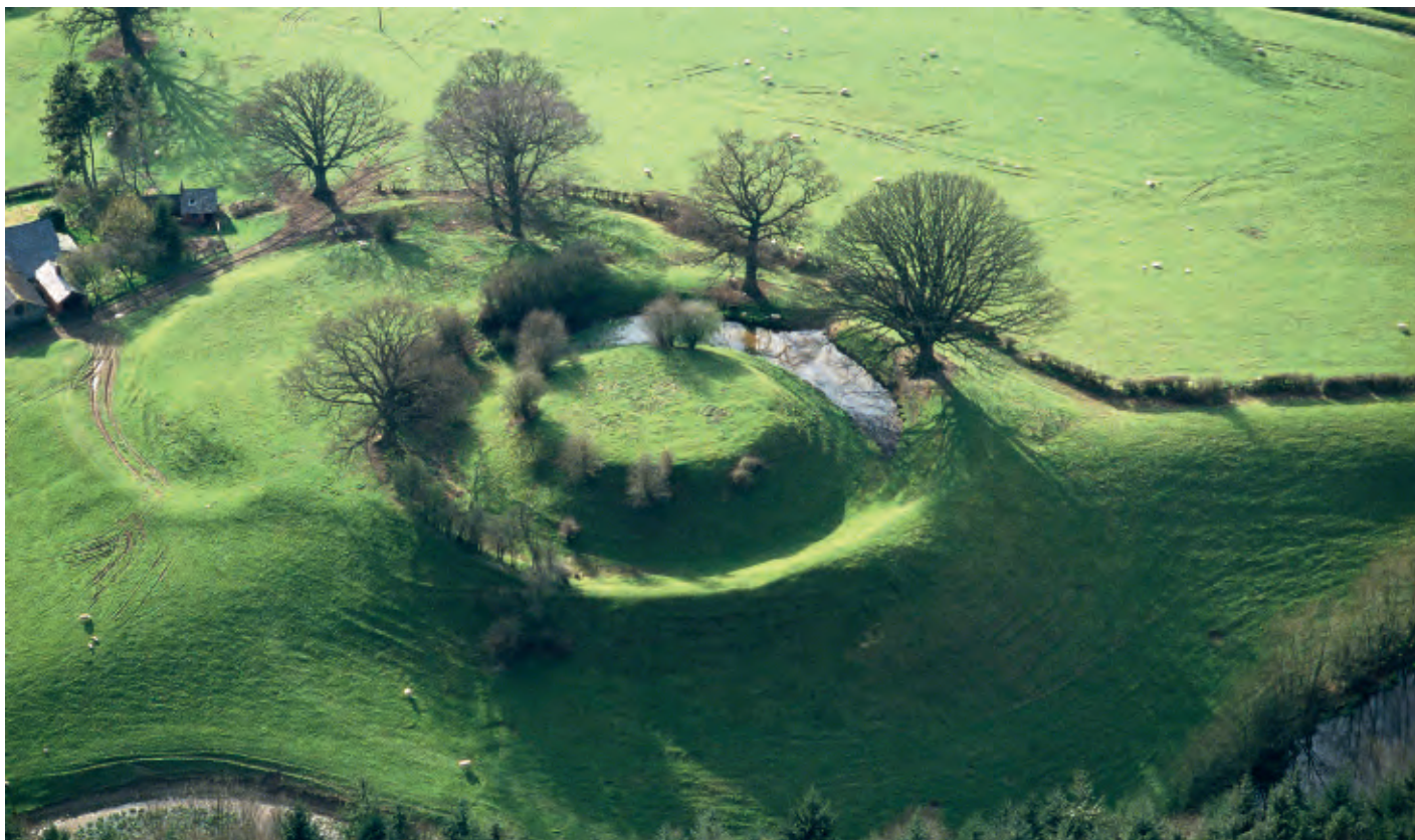
Figure 1. Owain Glyndŵr's home at Sycharth Castle, as it is today. Photo: Crown copyright, Royal Commission on Ancient and Historical Monuments of Wales.
