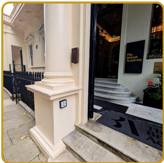
No. 10 Stairs and Bell with 8 steps.
