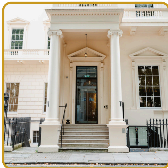
No. 11 Stairs with 9 steps.
