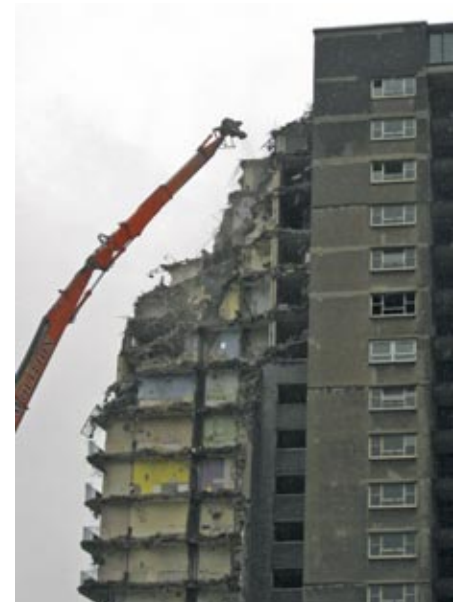
Tower block demolition in Glasgow
