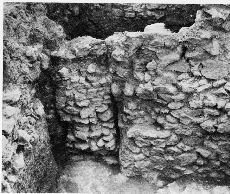
b. Blocked doorway of Room T 7 .
