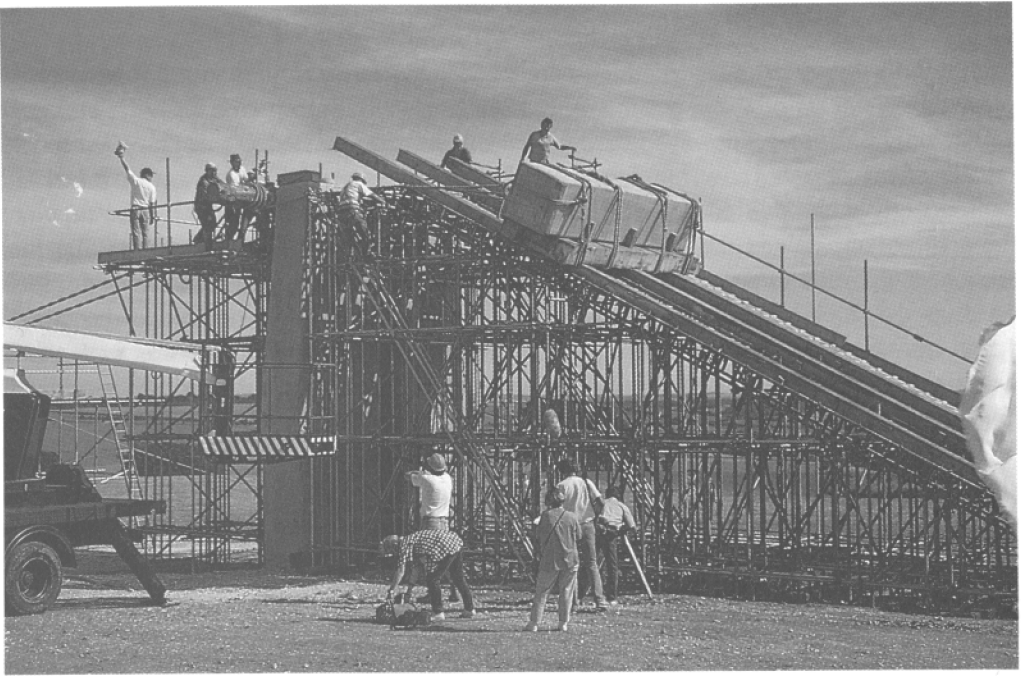
Figure 12. The use of a ramp to raise the lintel. (Copyright: Julian Richards.)
