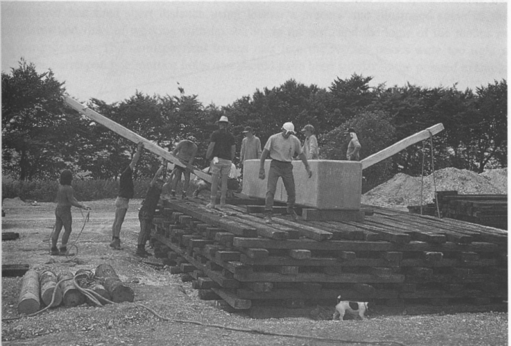
Figure 10. The use of the timber 'crib' and levers to raise the lintel. (Copyright: Julian Richards.)
