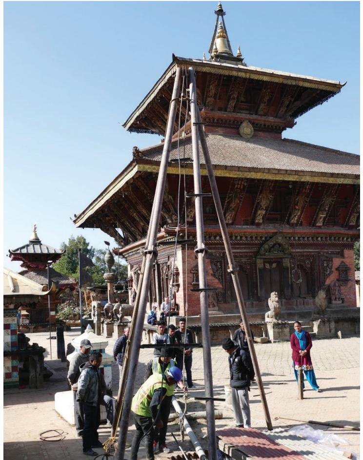
Geotechnical sampling next to the Changu Narayan Temple in Kathmandu’s World Heritage Site. PHOTO: DURHAM UNESCO CHAIR.
