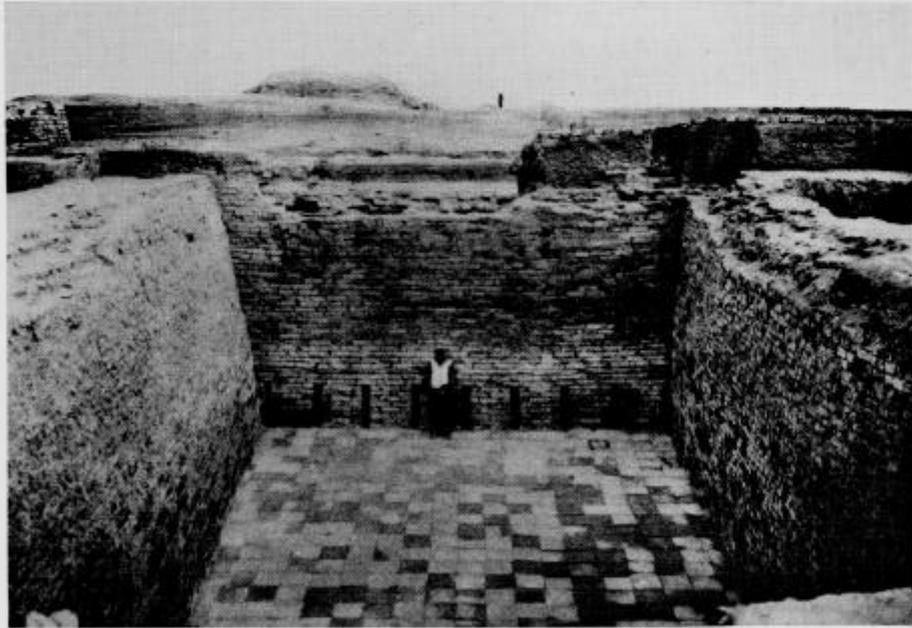
(b) Choga Zanbil. The brick-built reservoir showing the great tank and ducts connecting it with the inner basin.
