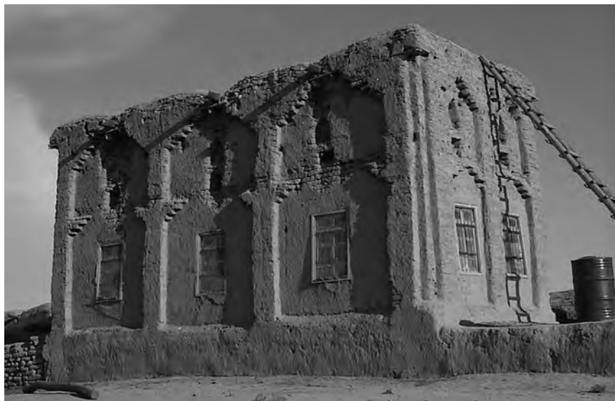
Figure 24. Mud-brick diwan in a village just south-east of Brak, a type of house built for the reception of visitors and now disappearing from the local landscape.
